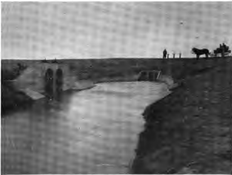
FIG. 111.—Lateral Headgates North Platte Valley, Nebraska.
